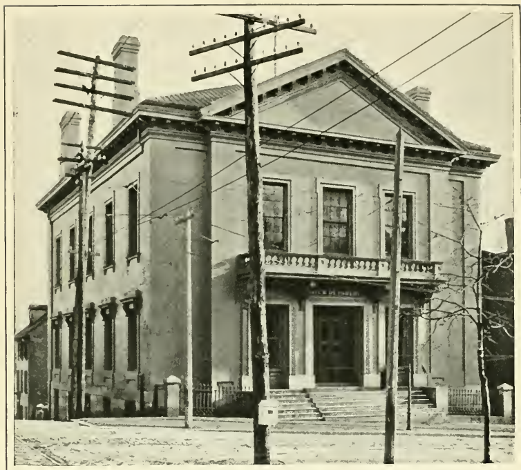
WILMINGTON POSTOFFICE AND CUSTOM HOUSE. 1855 TO 1897.
