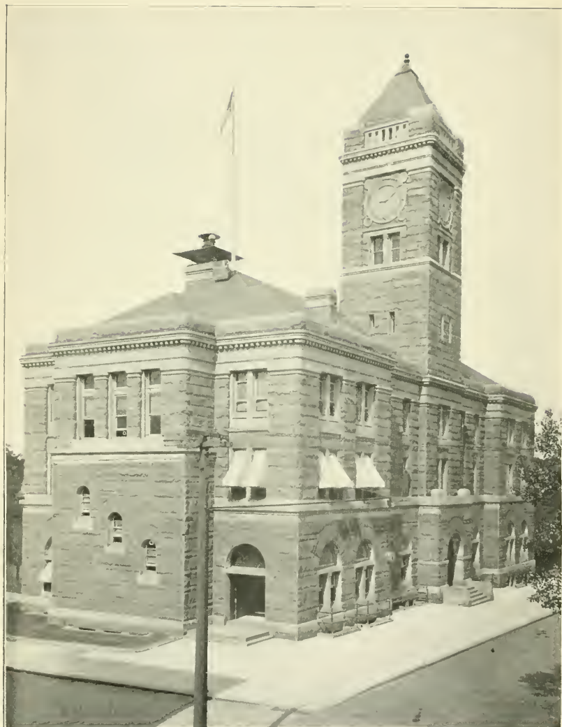
WILMINGTON POSTOFFICE AND CUSTOM HOUSE. A. D. 1897.
